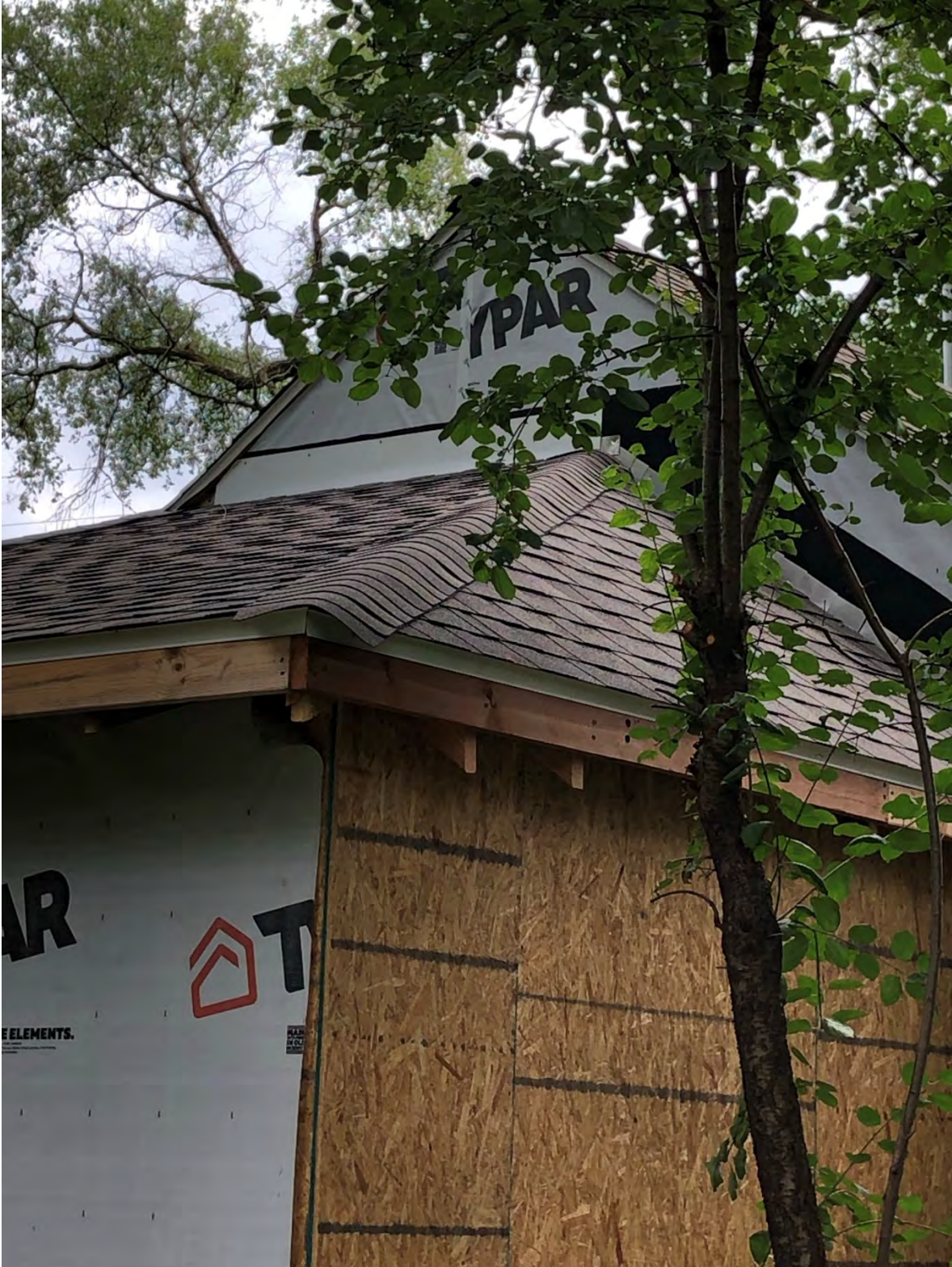
Detail of the altered lean-to addition and roofline. This picture was cited by the Building Official when he made the observation that it appeared that the exterior walls of the addition had also been raised in height.
