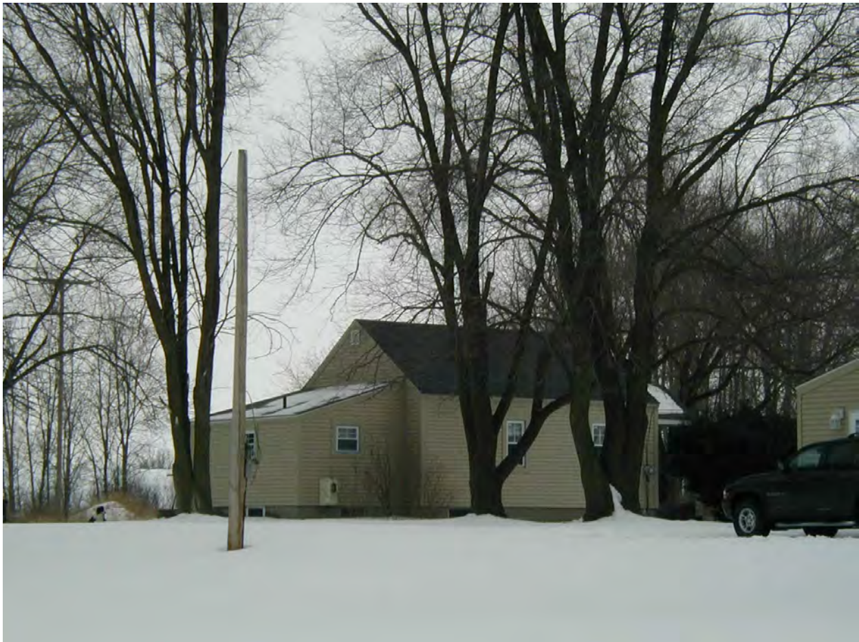
West side of the second dwelling showing the original lean-to roofline.
