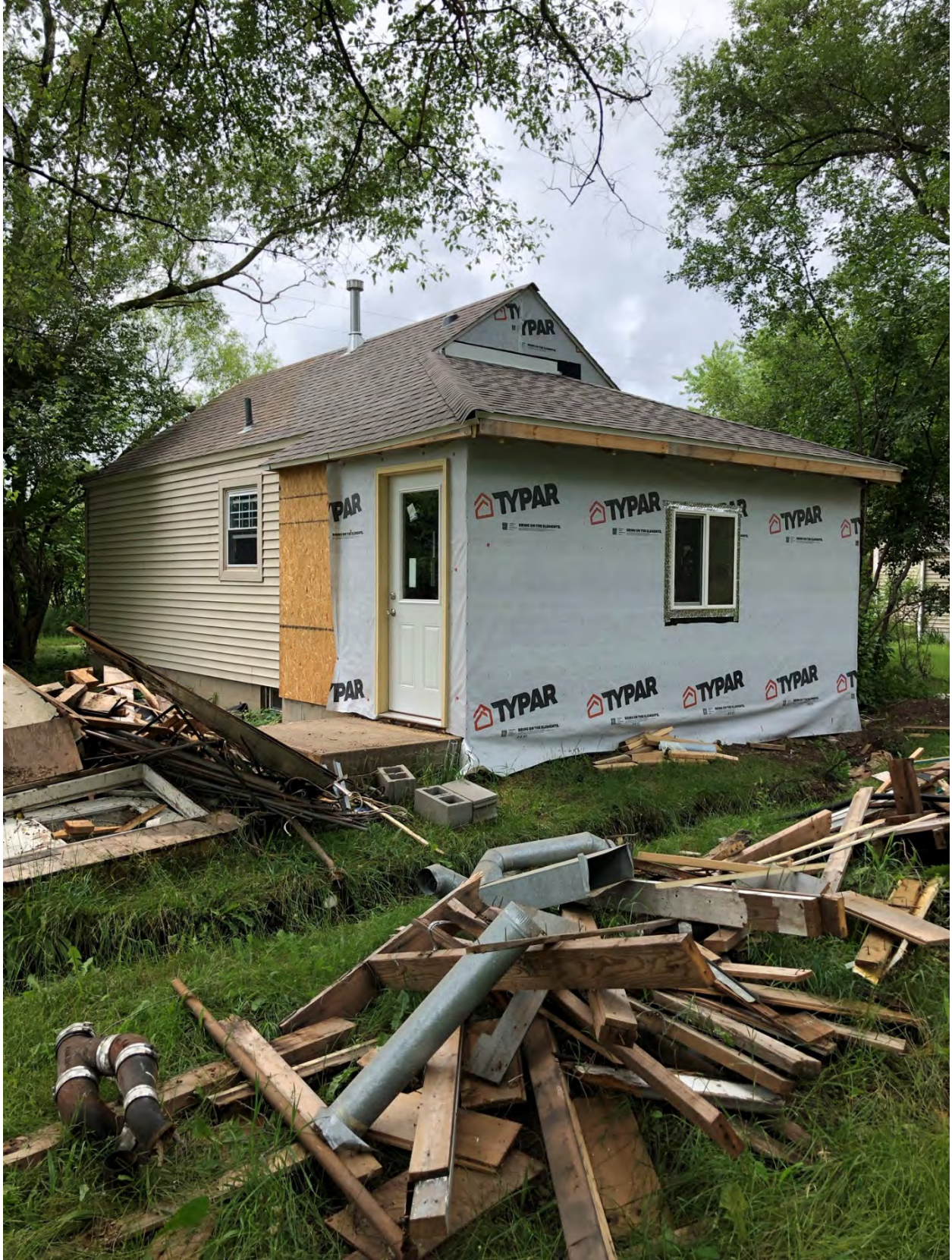
Building Official photo documentation of the unlawful construction activity. Note the steeper pitched roofline
