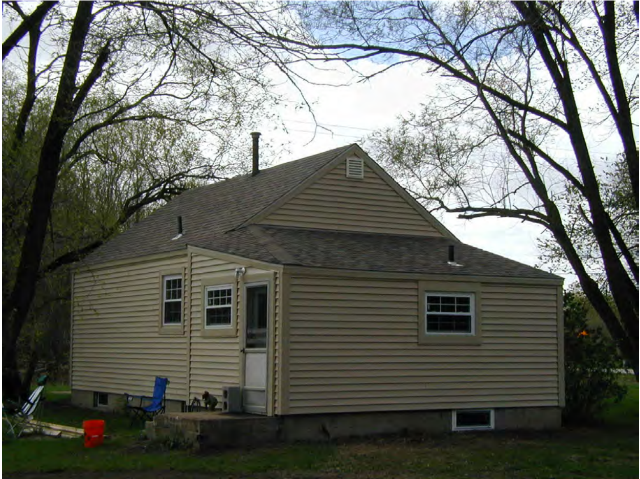
This is another view of the original character of the second dwelling from the Twp. Assessor's database. Note the low height of the rear wall in relation to the side entry door, and the low pitch of the original roofline.
