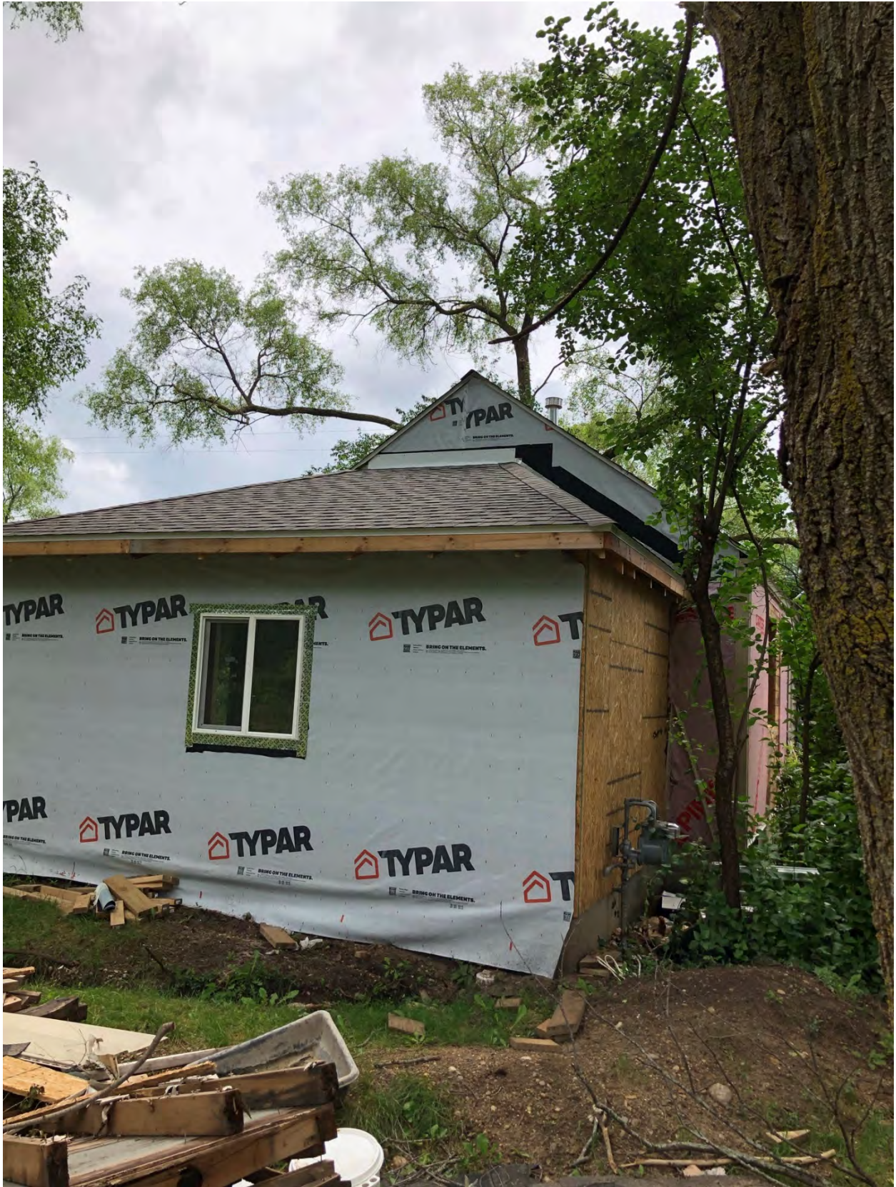
Second view of the lean-to addition as altered and enlarged in interior volume.
